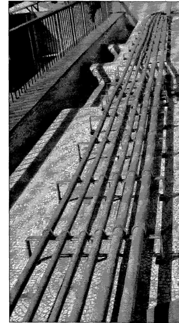
TERRACE FLOOR CLAMP FIXING AT SITE
